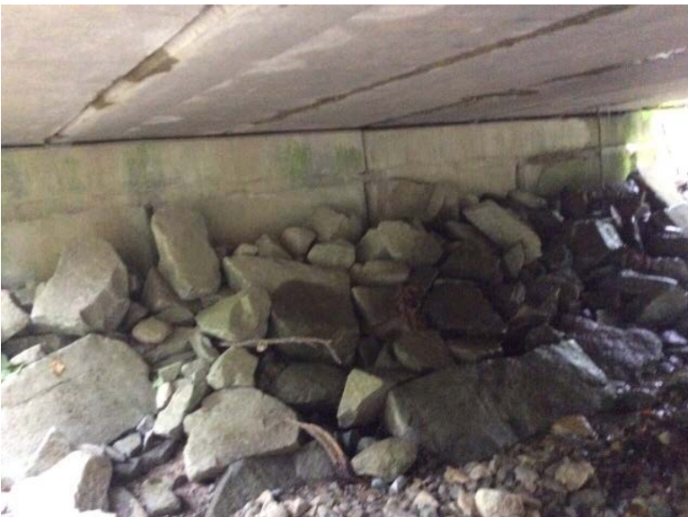
Left Bank Abutment when facing downstream
