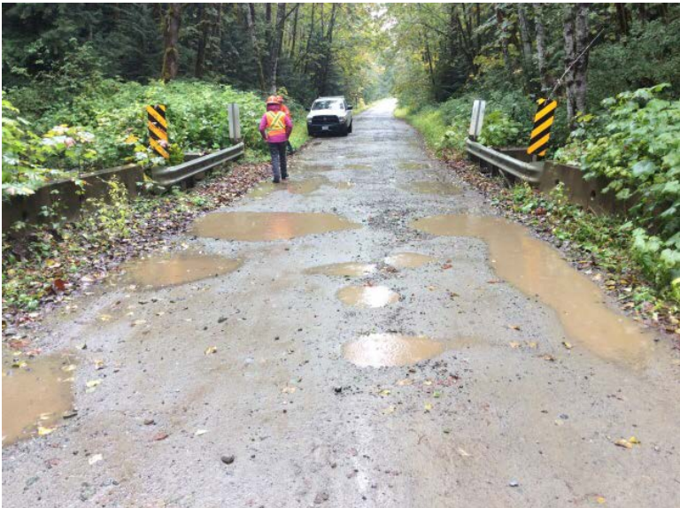
Approach from Right Bank when facing downstream
