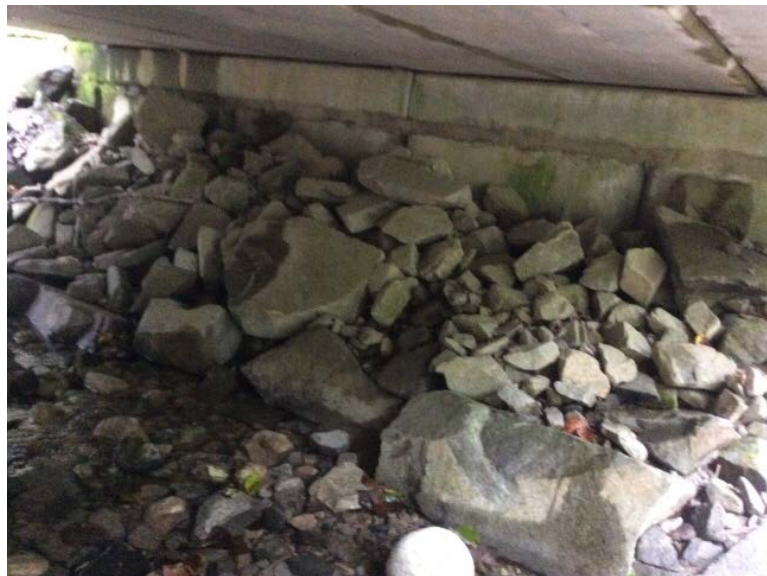
Right Bank Abutment when facing downstream
